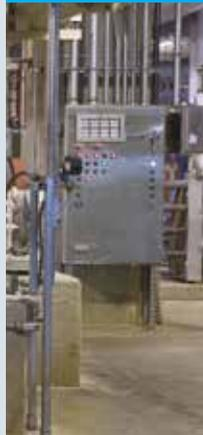
Remotely monitoring and controlling pumps, motors, conveyors, valves, packaging and assembly lines over wireless networks reduces manpower requirements; decreases costs through the precise control of operations; maintains continuous monitoring and control of processes; communicates malfunction warnings and enables an immediate response to system inconsistencies from a central location.
