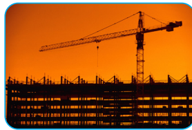
UNCABLED WORK SITES
